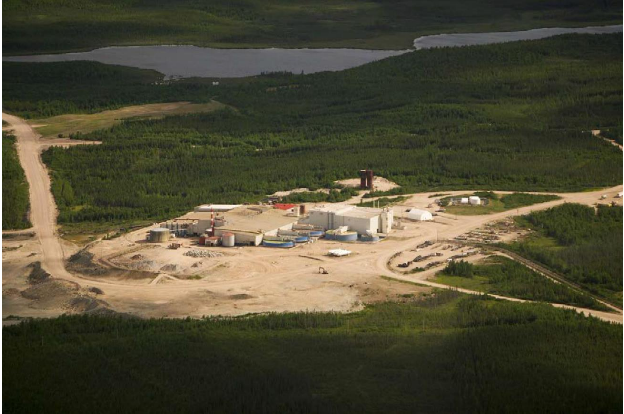
Figure 4: Aerial View of the Mill at Rabbit Lake (CNSC CMD H7-1, 2023)
