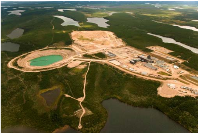
FIGURE 2: In-pit disposal of tailings
