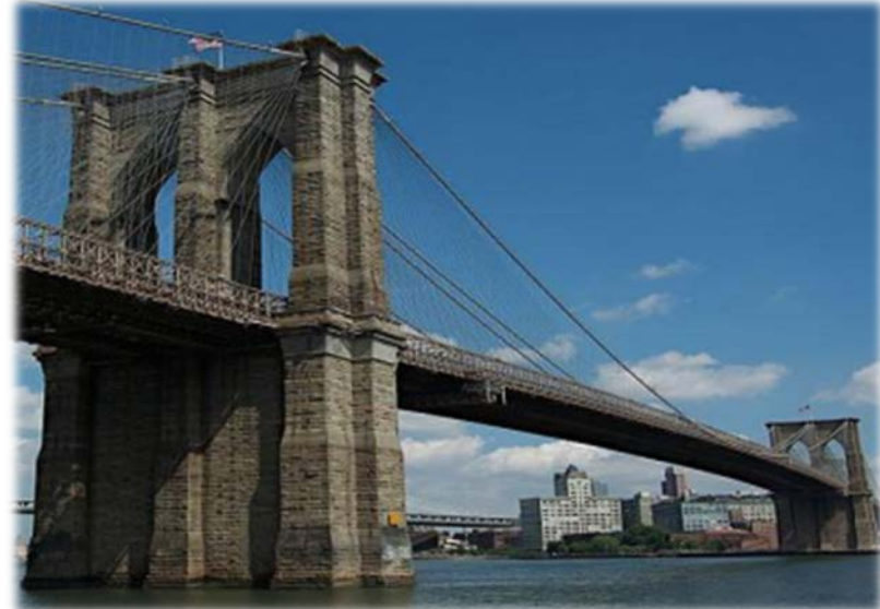
Brooklyn Bridge, New York City
